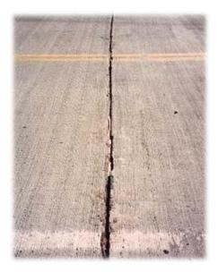
Repair: easy to remove the seal and refill
