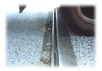
Repair: usually replace the entire seal, leakage areas filled with adhesive, debris removed
