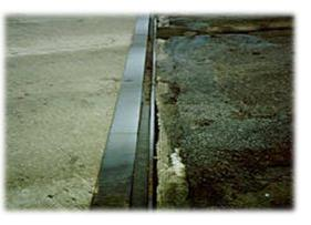
Repair: Replacement, debris removal, re-welding specific locations
